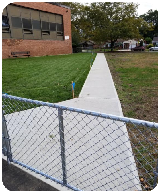
New Willow walkway from front to rear of building improves safety
